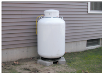
Lewiston 420 tank install with piping
