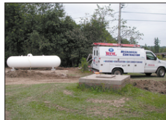
Sabattus 1000 above ground tank install with underground piping
