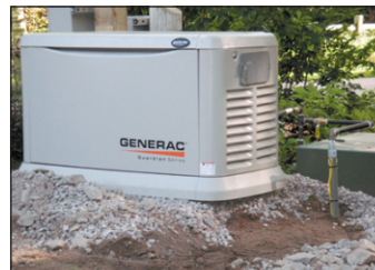
Topsham Residential generator install with underground piping
