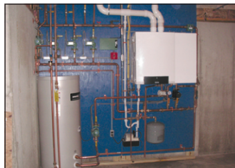
Lewiston Residential high-efficiency heating system installation
