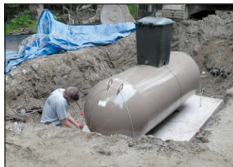
Auburn 500 underground tank install
