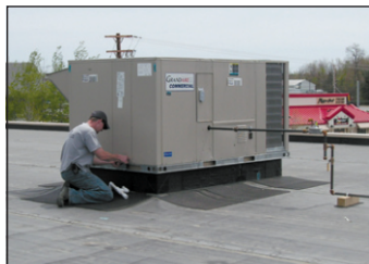
Rockland Commercial roof top install with complete ductwork
